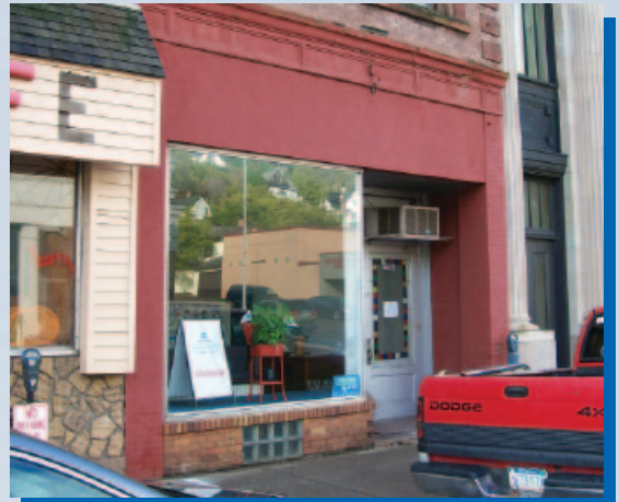
Last November KCF moved into its new home at 236 Quincy Street in Hancock. A new front wall design is in the works.
